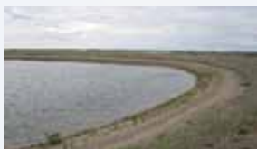
Tuktoyaktuk Raw Water Reservoir
