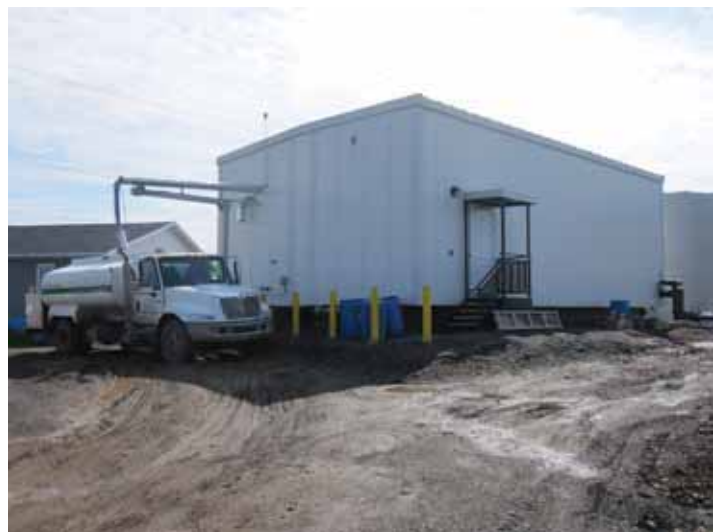
Aklavik Water Treatment Plant
