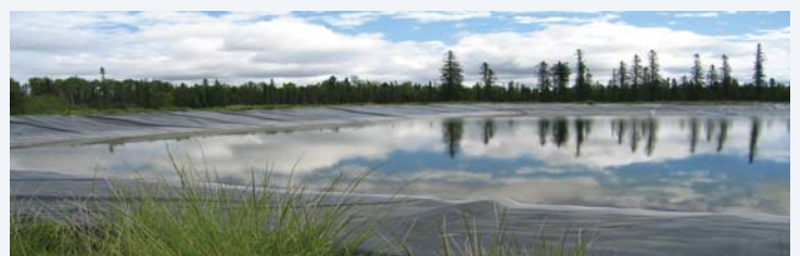
Raw Water Reservoir in Jean Marie River
