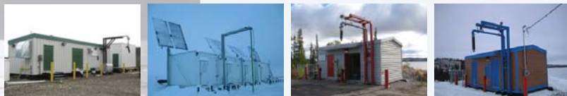
Water Treatment Plants (Left to Right): Tulita, Colville Lake, Gamèti, Wekweèti
