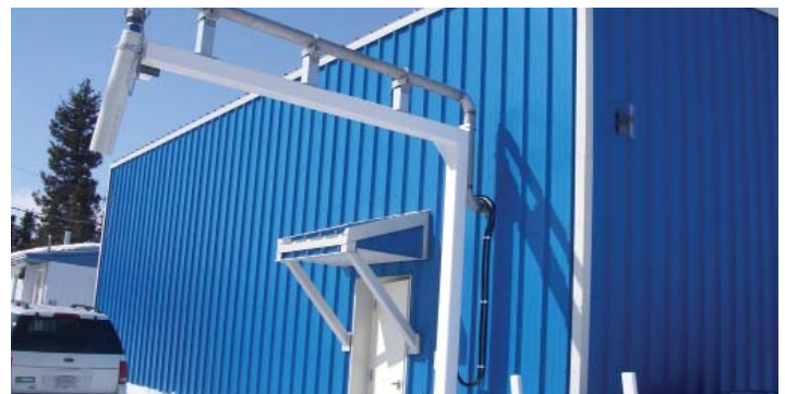
Behchokò (Edzo) Water Treatment Plant
