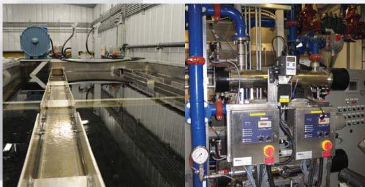
New Water Treatment Plant in Behchokò (Edzo) (Left) UV Reactor in the Déljné Water Treatment Plant (Right)
