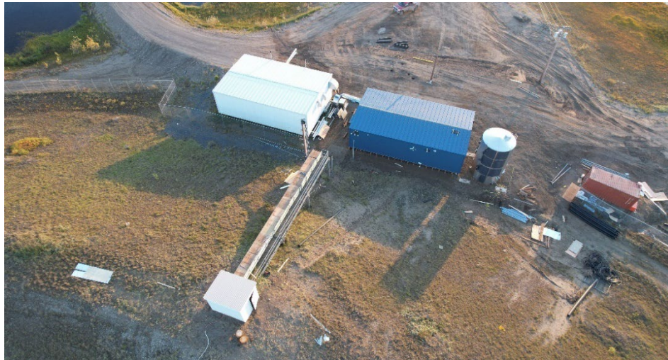
Aerial photo of Tuktoyaktuk's new water treatment plant in blue beside the current plant.
