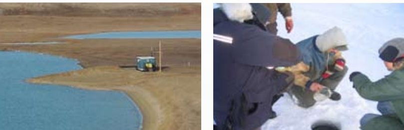
Picture on the left: Paulatuk Water Treatment Plant on New Water Lake Picture on the right: Tuktoyaktuk Foreman, Peter Nogasak, taking samples from the raw water reservoir.
